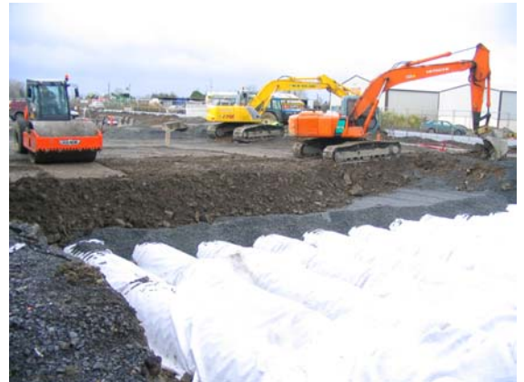
360 m 3 DRAIN-MAX Tunnel-System in Irland
